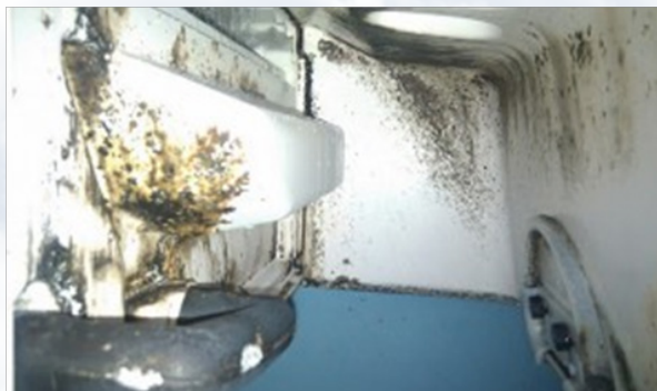
Ice Machine covered in slime & mold.
